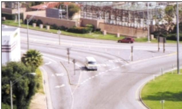
Flare on an entry to a roundabout is the widening of an approach to multiple lanes to provide additional capacity and storage at the yield line. *Long Beach, CA*
