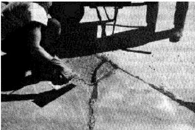
Figure 4. Finishing a patch containing an active crack.
