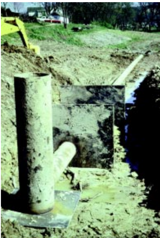
Figure 22 Drop-inlet pipe spillway with antiseep collar
