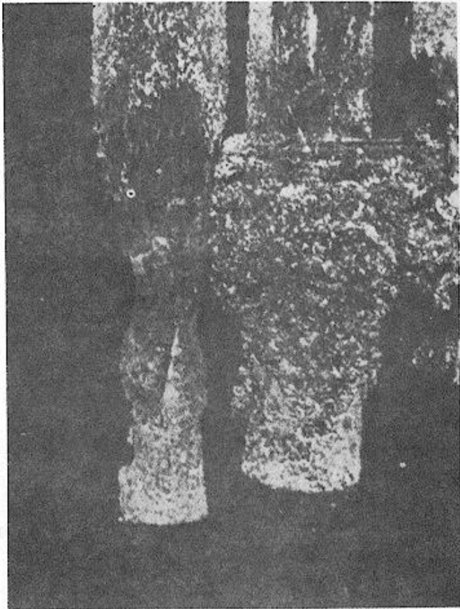
Figure 2-2. Destruction of wooden piers by marine borers.
