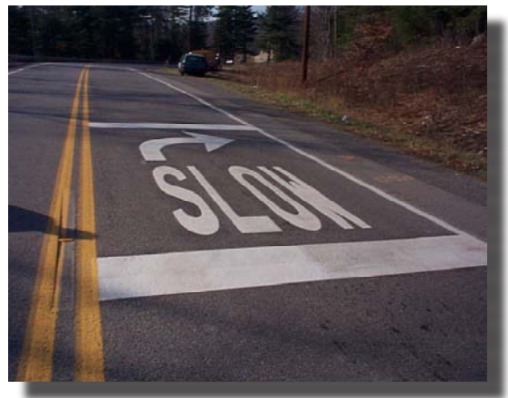
PennDOT curve advance marking.
