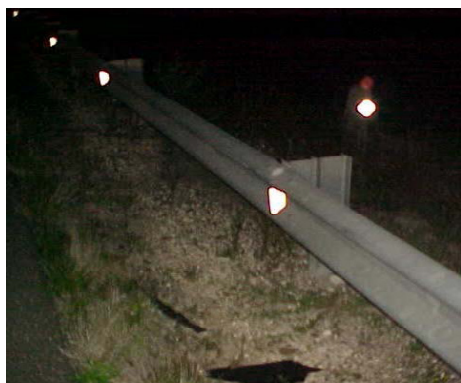
Installation of reflectors on W-beam guardrail.
