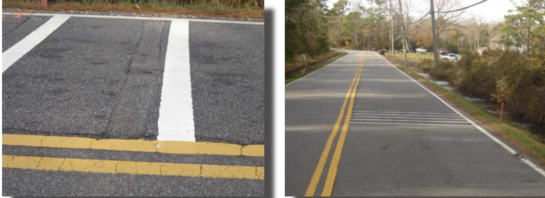
For this RRS application a set of 5 grooves and painted lines were placed 200 ft before the curve.
