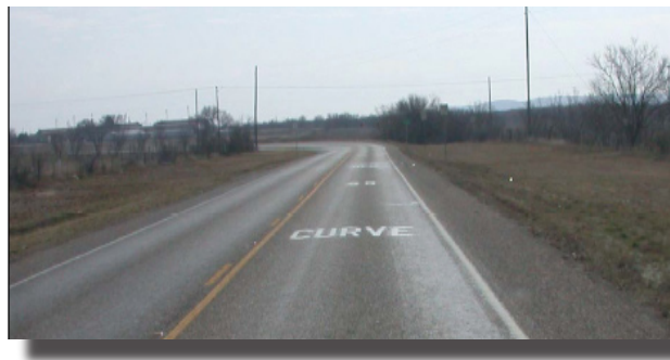
Speed-limit advisory pavement marking.
