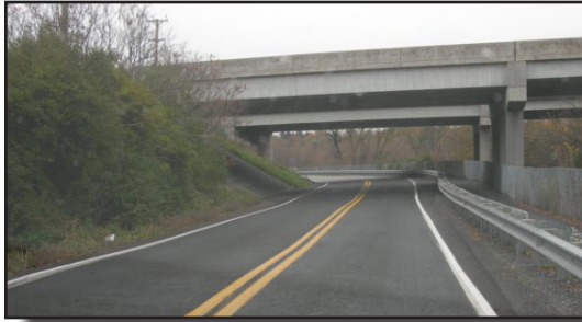
Centerline and edge line for two-lane road.
