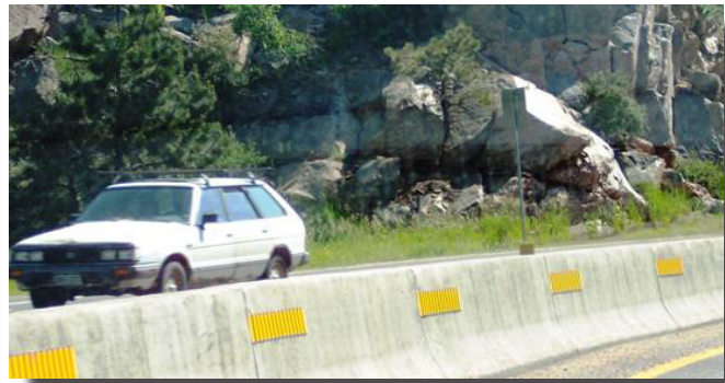
Reflective sheeting shaped to provide linear reflectorization.
