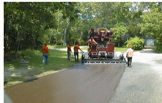
Application of skid-resistant pavement surface in curve.
