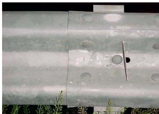
Installation of reflectors on W-beam guardrail.
