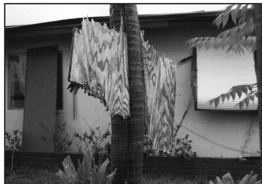
A plywood missile lodged in a palm tree, Hurricane Andrew
