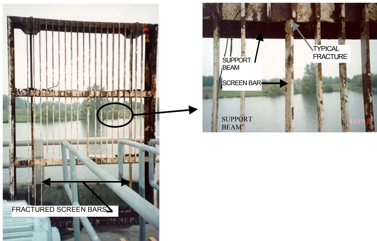
Figure 8-10. Fractured screen bars on dam intake trashrack
