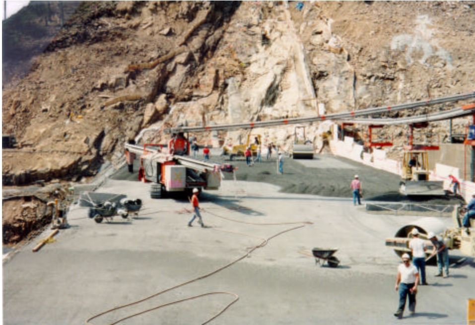
Figure 6-1. Conveyor system with self-propelled crawler-placer
