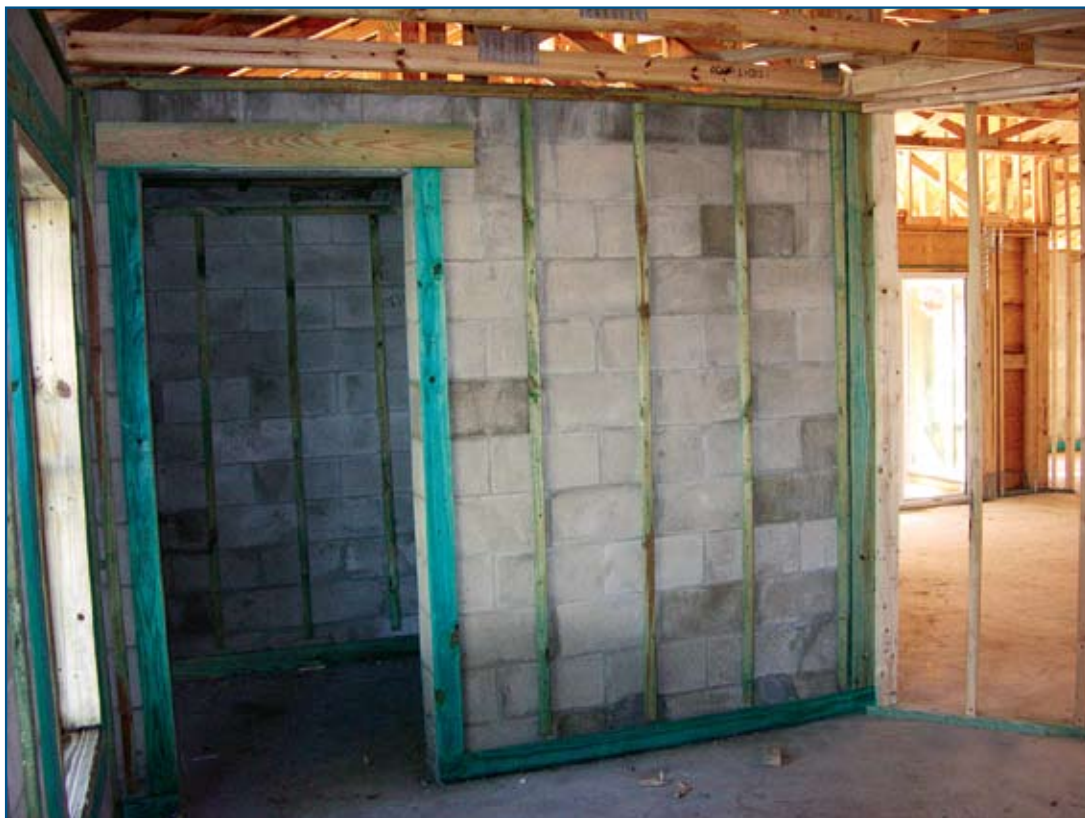
Figure II-6. View of an in-home safe room under construction. The CMU walls of this safe room are fully grouted and are reinforced, vertically, with steel reinforcing bars from the foundation to the concrete roof deck (New Smyrna Beach, Florida).
