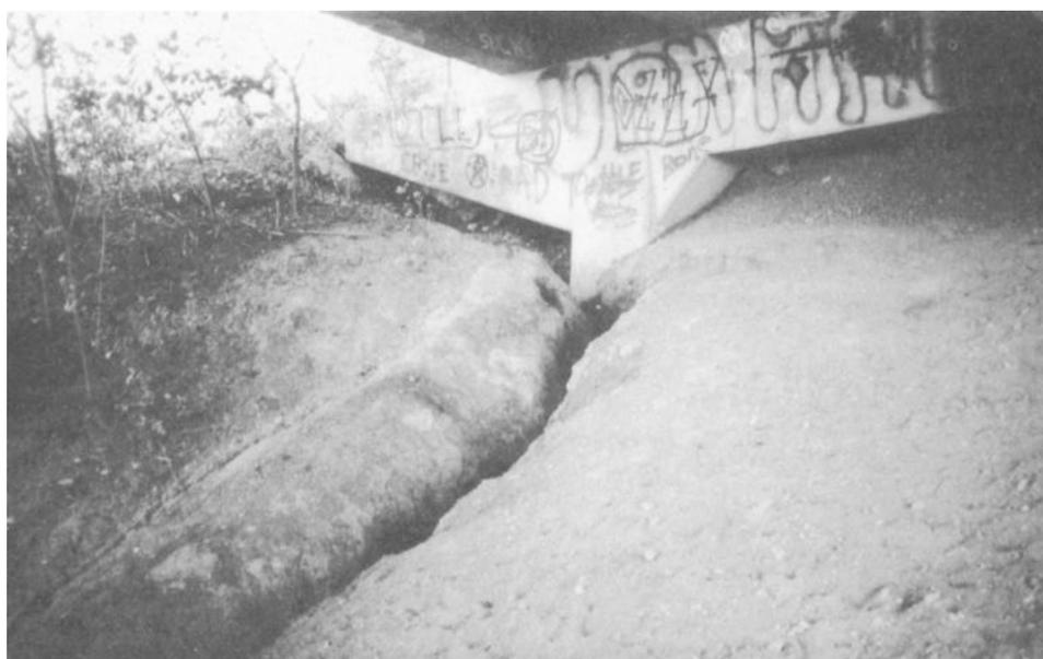
Figure 5-25. Embankment erosion due to improper drainage. (Sheet 2 of 2)
