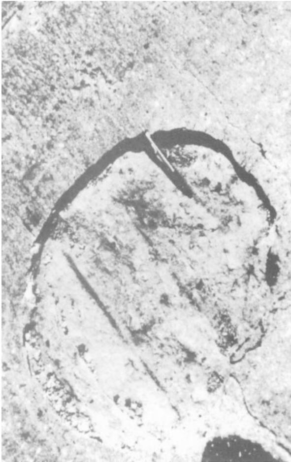
Figure 5-8. Large spall.
