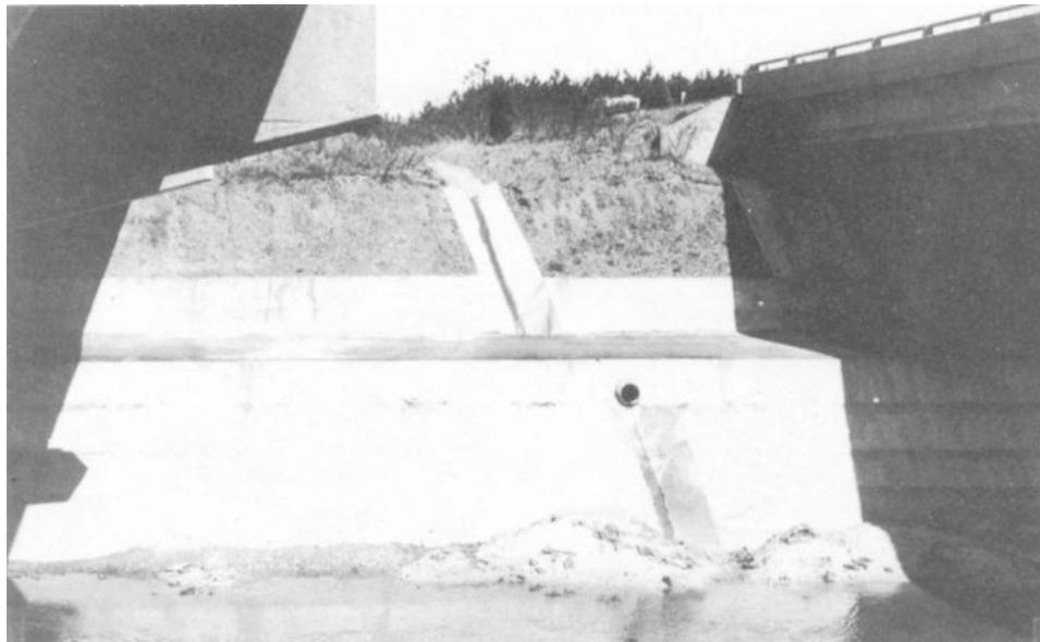
Figure 5-38. Concrete slope protection.
