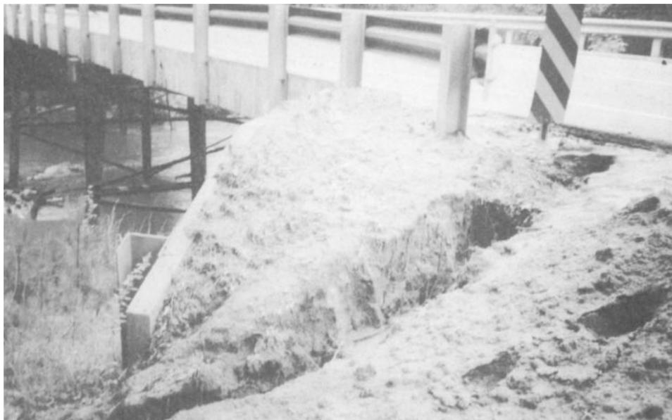
Figure 5-25. Embankment erosion due to improper drainage. (Sheet 1 of 2)
