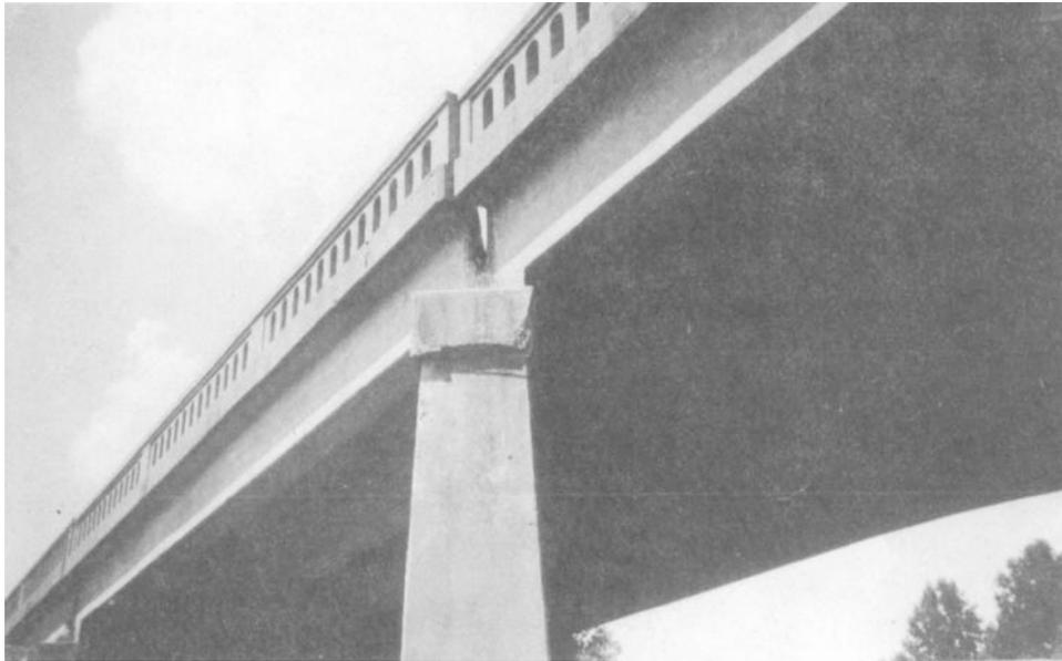
Figure 5-21. Differential pier movement causing superstructure movement.
