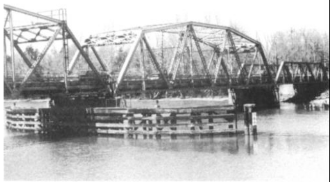
Figure 3-19. Timber bent fenders.
