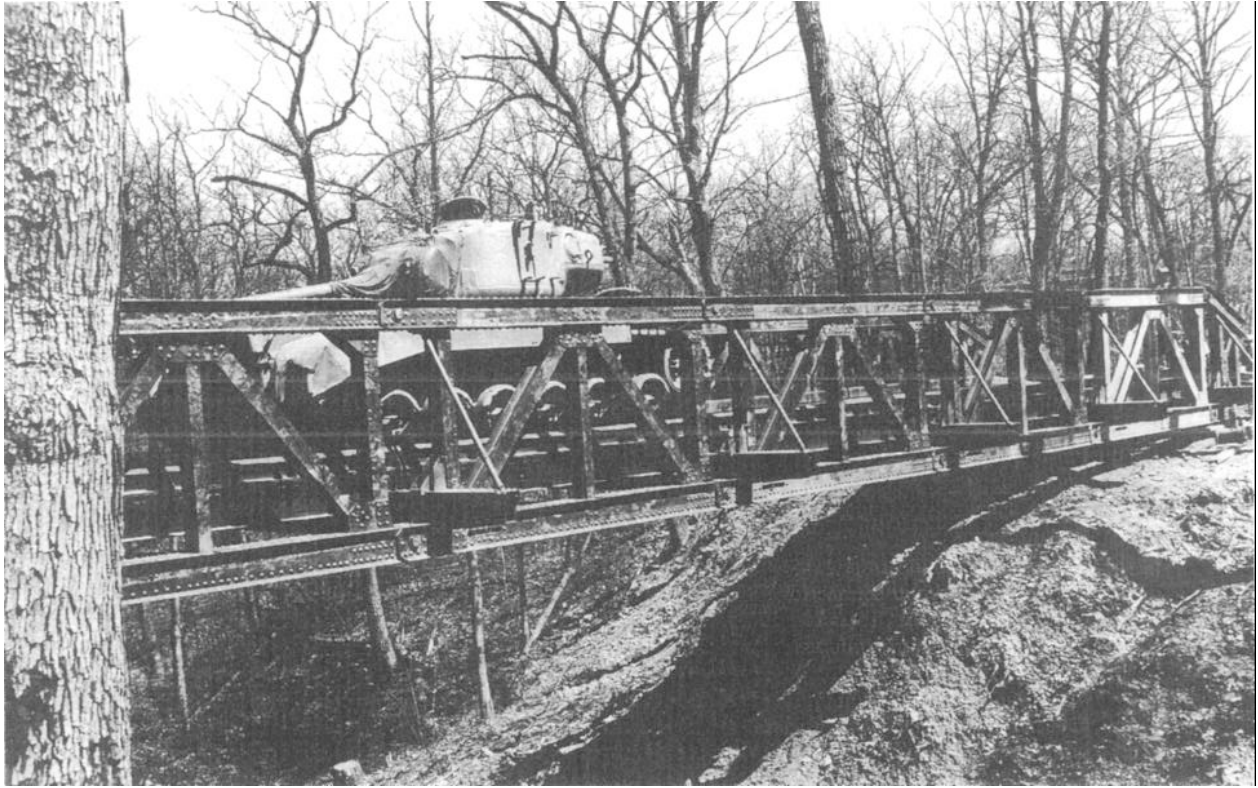
Figure 2-8. T6 aluminum fixed bridge.
