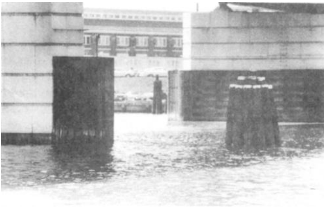
Figure 3-18. Timber pile cluster dolphins and timber fenders.
