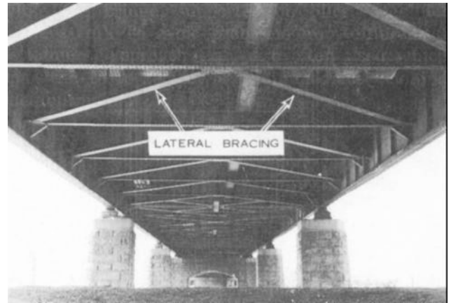
Figure 3-9. Bracing. (Sheet 2 of 2)
