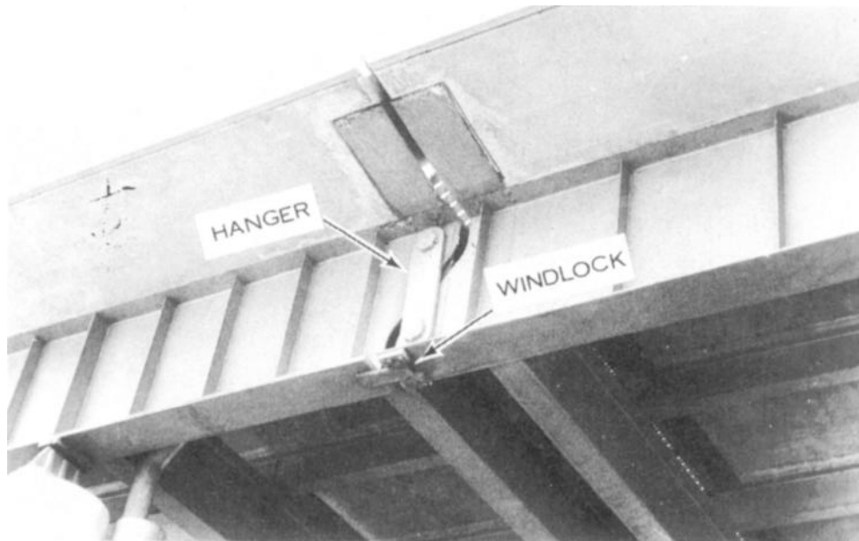
Figure 3-14. Pin and hanger connection.
