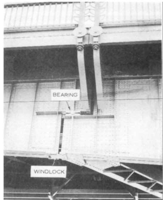
Figure 3-13. Bearing support for a suspended span.
