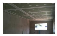
This is a new section requiring floors to be covered with a minimum ½ inch gypsum board or 5/8 inch wood structural panel on the underside. Exceptions are provided for fire sprinklers and certain crawl spaces.
