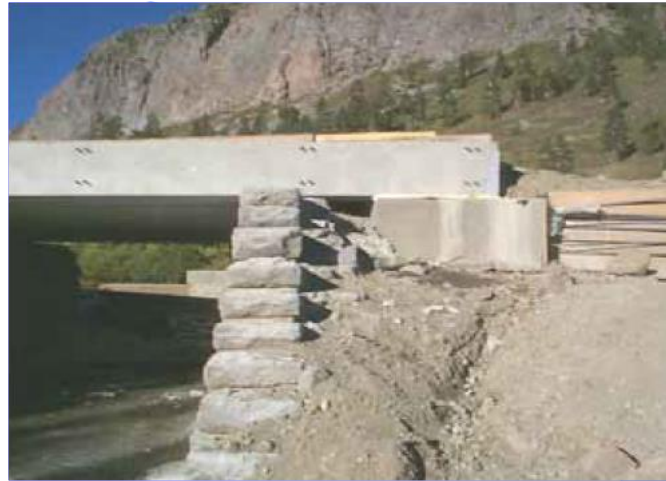
Figure 32. GRS abutment behind historic stone abutment.
