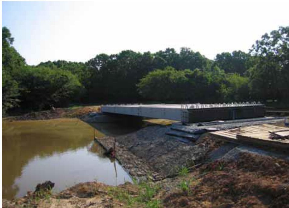
Figure 35. Concrete box bridge on GRS abutment in Ouachita wildlife refuge.
