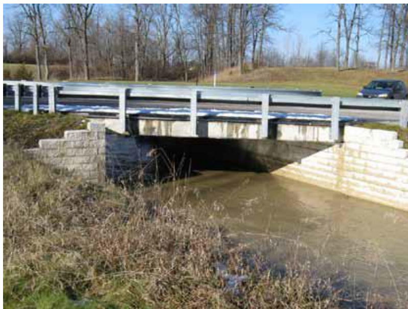
Figure 17. Vine Street Bridge.
