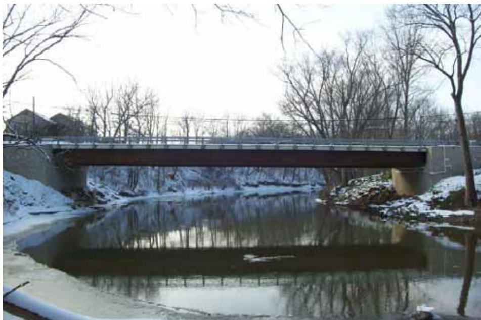
Figure 25. Tiffin River Bridge.
