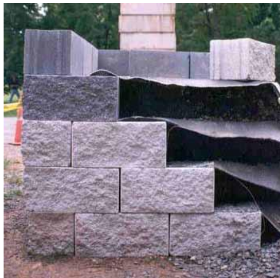
Figure 6. Photo. Cut-away of GRS mass.
