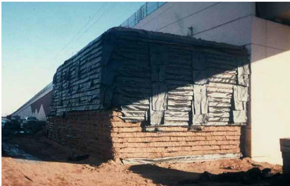
Figure 8. Photo. Internally supported GRS structure.
