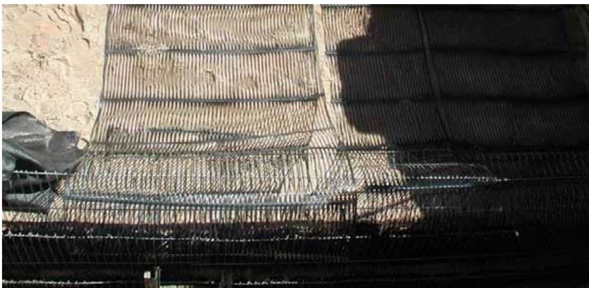
Figure 4. Photo. MSE extensible reinforcement (geogrid).
