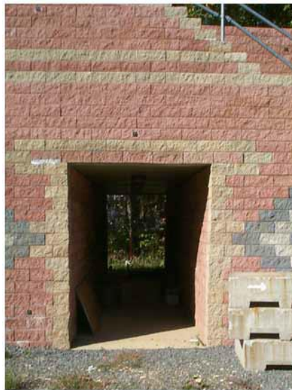
Figure 29. Close-up of GRS-IBS tunnel at TFHRC.
