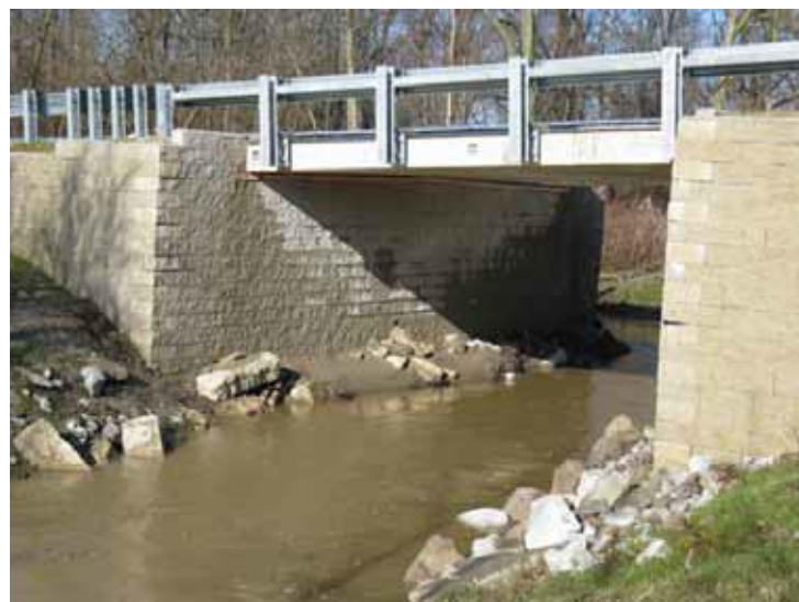
Figure 21. Huber Road Bridge.
