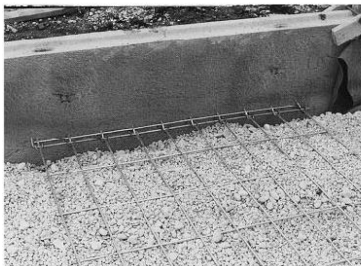
Figure 3. MSE inextensible reinforcement – wire mats
