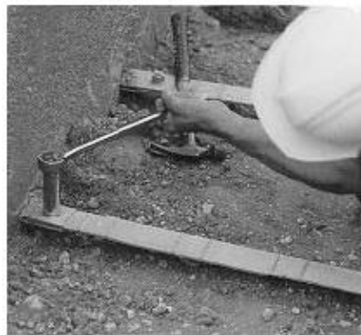
Figure 2. MSE inextensible reinforcement—steel strips.
