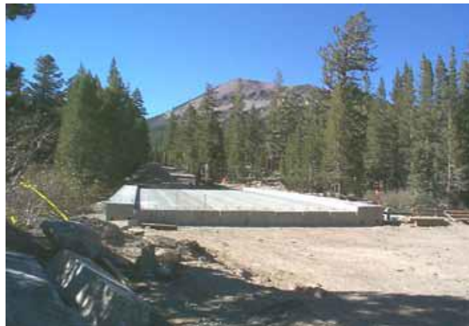
Figure 33. Concrete box bridge on GRS abutment in Mammoth Lake, CA.
