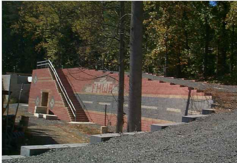
Figure 28. GRS-IBS tunnel at TFHRC.
