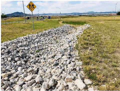
Figure 5 – Riprap Lining
