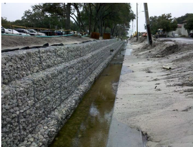
Figure 16 – Gabion Baskets (Courtesy of R.H. Moore & Associates)
