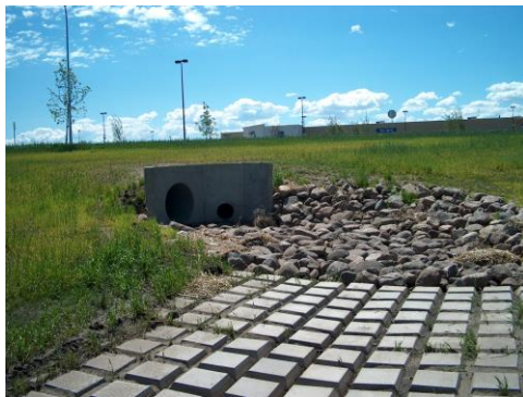
Figure 8 – Cabled Concrete Blocks
