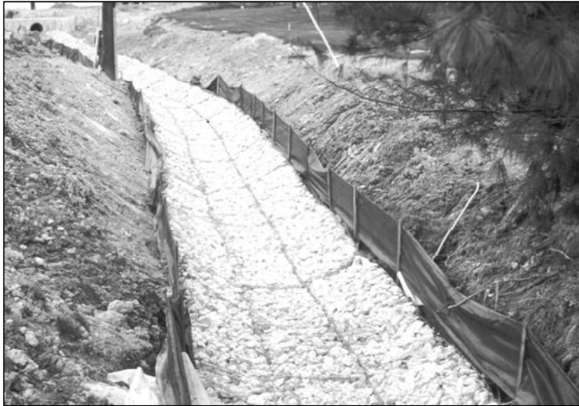
Figure 6. Wire-Enclosed Riprap
