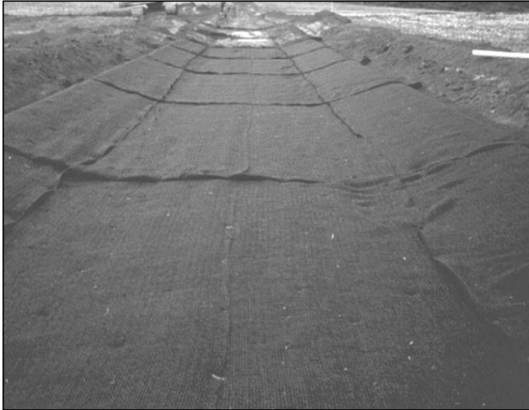
Figure 7 – TRM in channel
