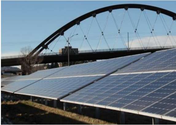
Figure 8. DFC Solar Array Near Bridge
