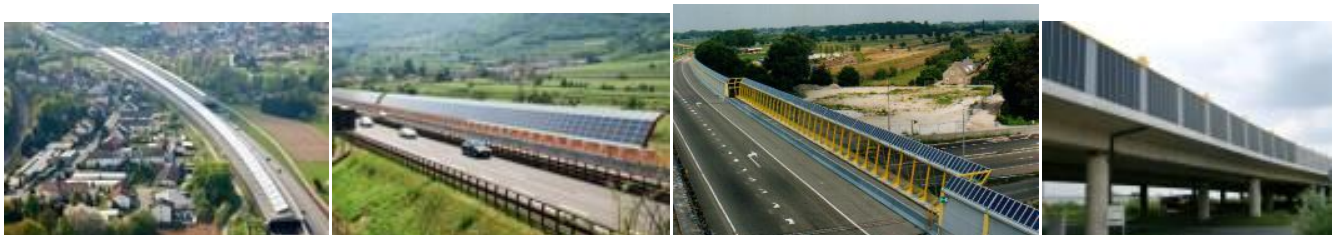
Figure 1. PV Arrays in Noise Barrier
