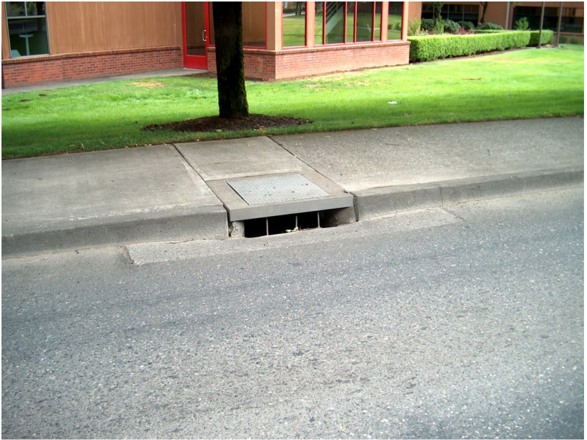
Figure 3 – Short Curb Opening Inlet
