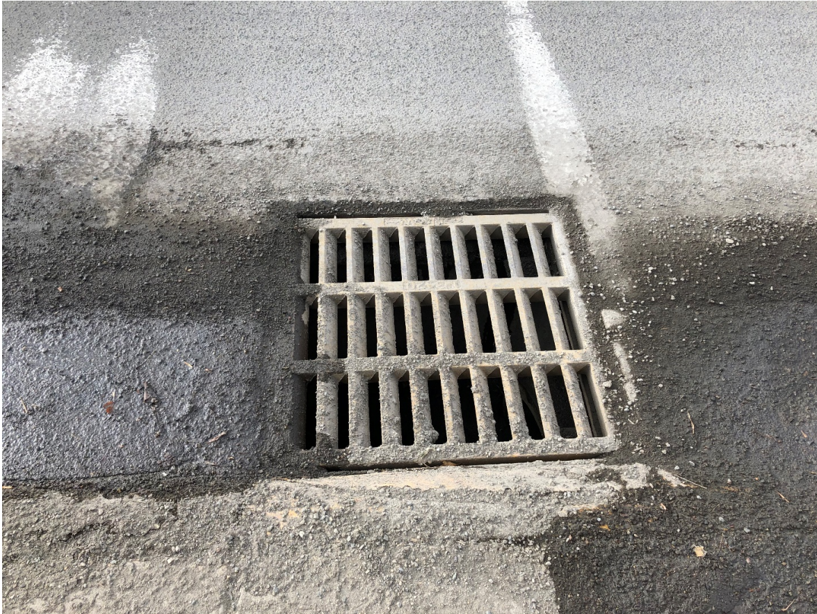
Figure 2 – Vane Style Inlet
