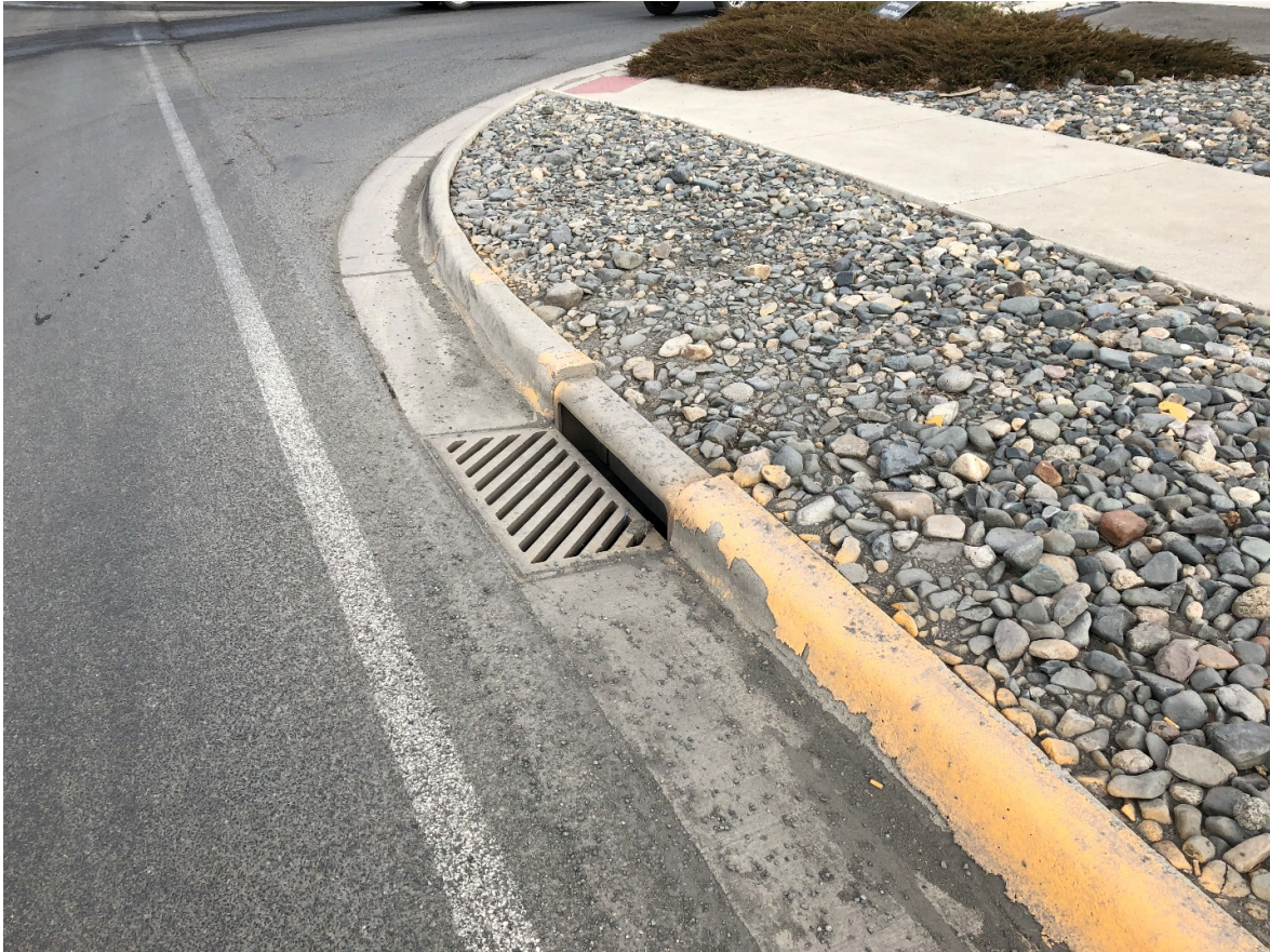
Figure 5 – Combination Inlet
