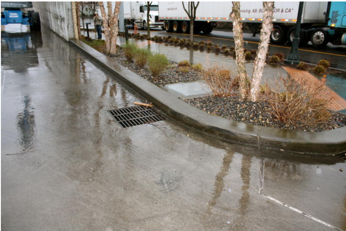
Figure 1 – Grate Inlet
