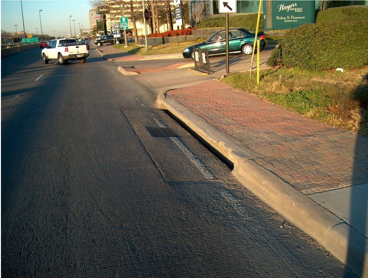
Figure 4 – Long Curb Opening Inlet
