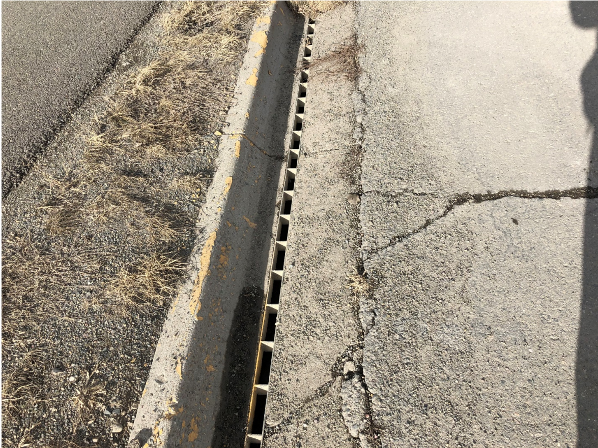
Figure 6 – Slotted Drain
