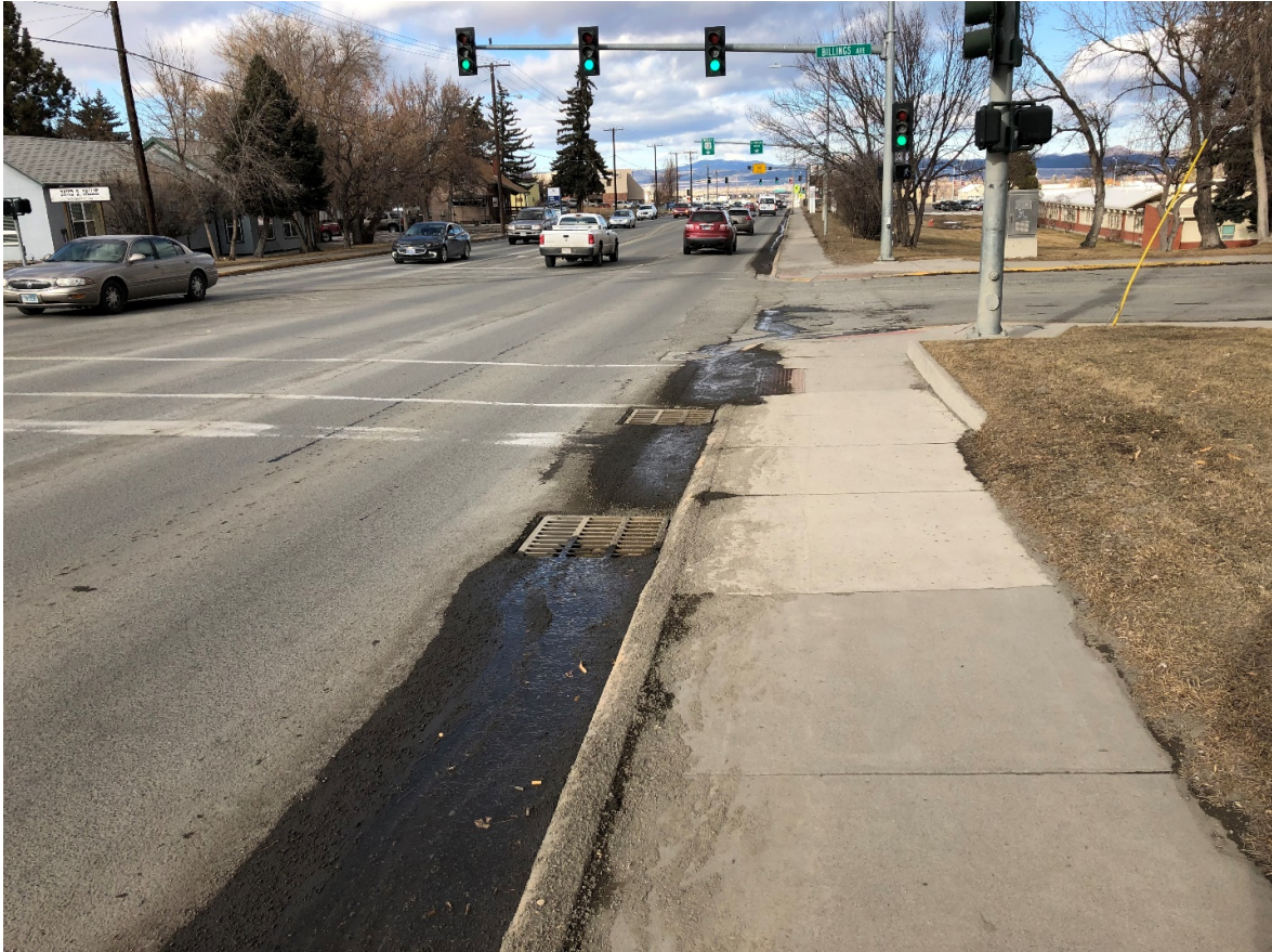
Figure 17 – Double inlets, spaced 8 feet apart
