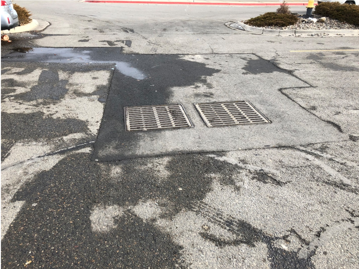
Figure 20 – Multiple grates in a parking lot
