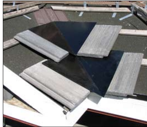
Figure 2. Special valley flashing to avoid debris accumulation between and below tiles (photograph courtesy of MonierLifetile).
