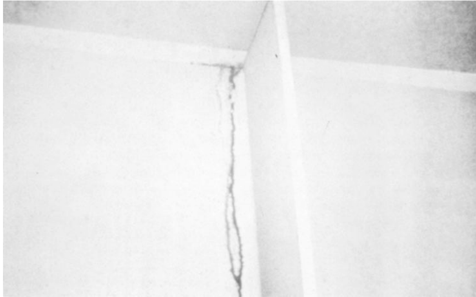
Figure 5-12. Rust stained crack in steel girder.
