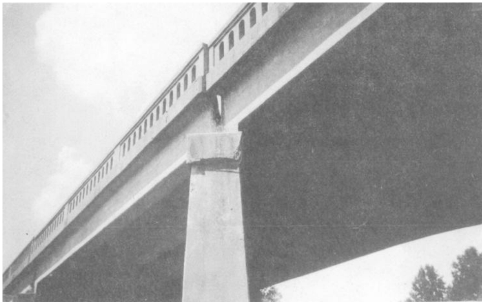
Figure 5-21. Differential pier movement causing superstructure movement.
