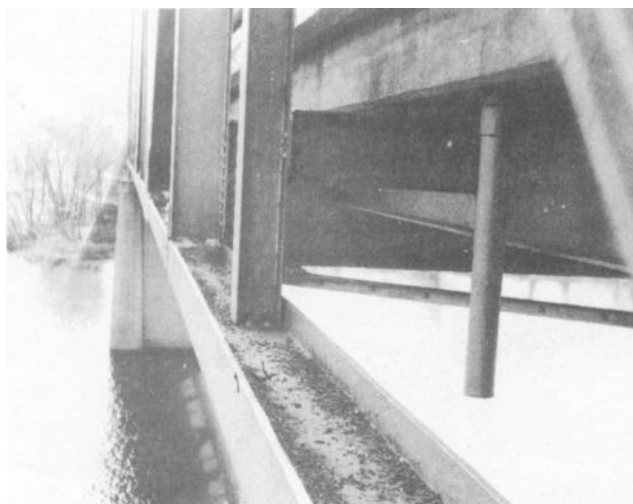
Figure 8-23. Lower chord of a riveted truss.
