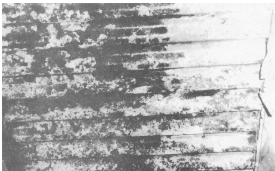
Figure 8-29. Rusty stay-in-place forms underneath a concrete deck.
