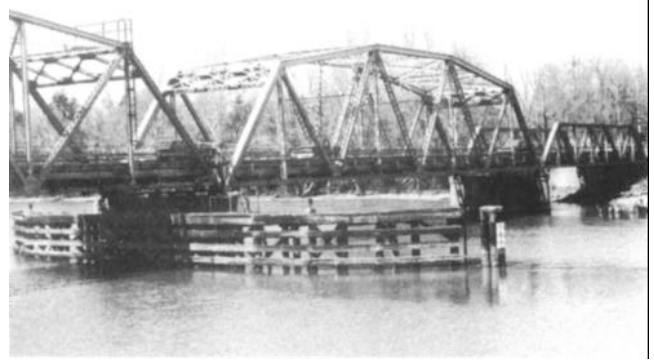
Figure 3-19. Timber bent fenders.
