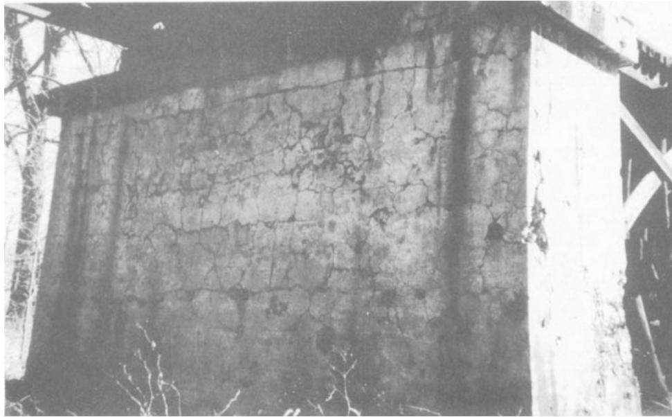
Figure 5-1. Pattern or map cracking on a pier.
