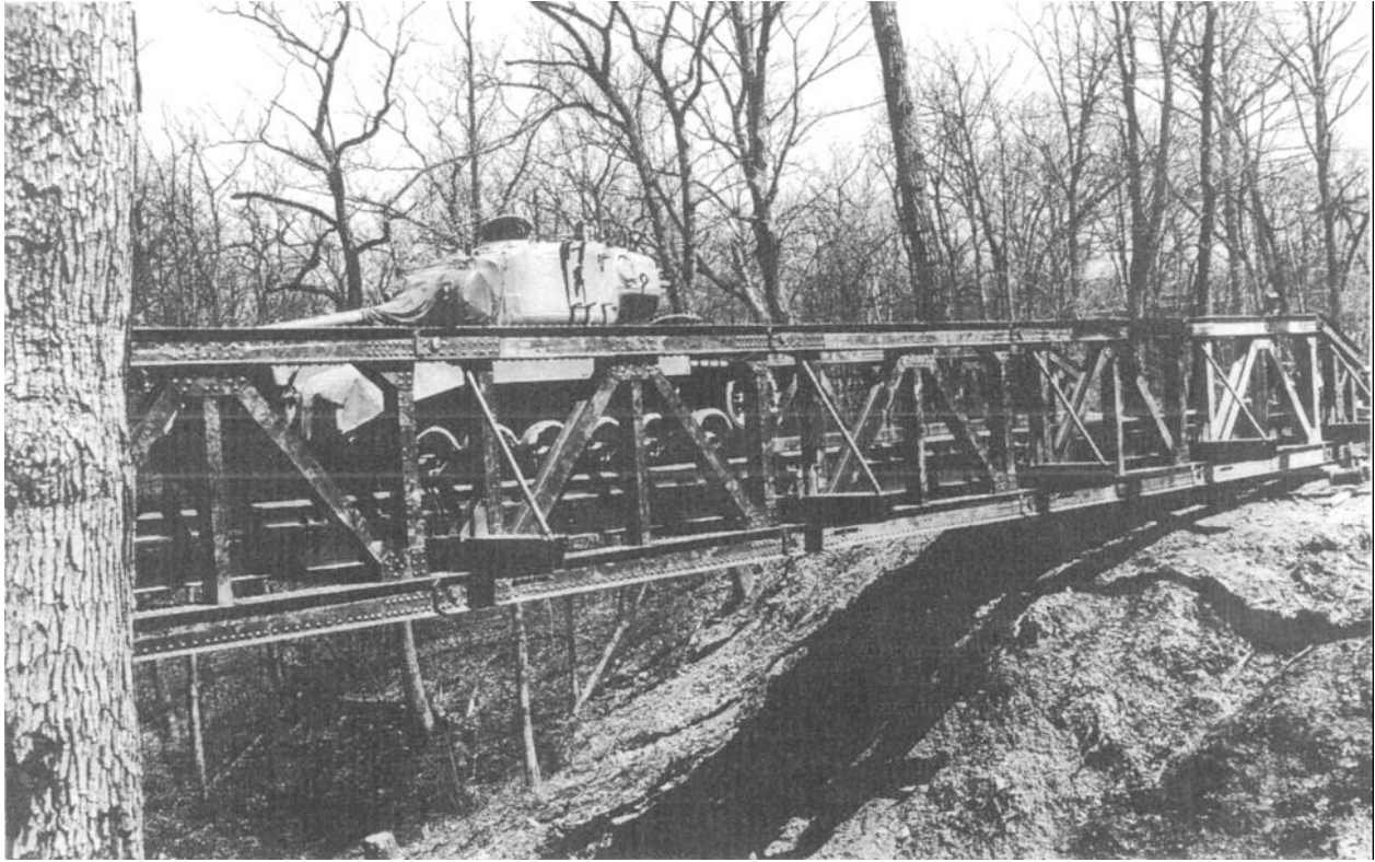
Figure 2-8. T6 aluminum fixed bridge.
