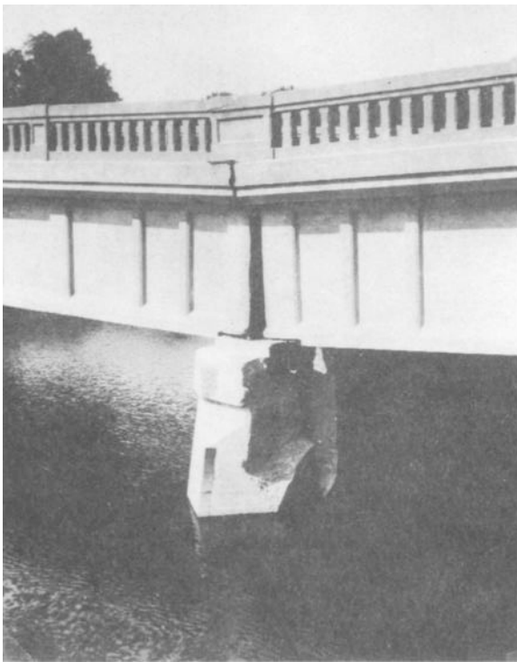
Figure 5-22. Movement due to scour.
