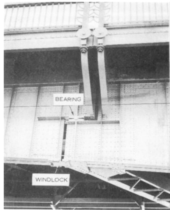
Figure 3-13. Bearing support for a suspended span.
