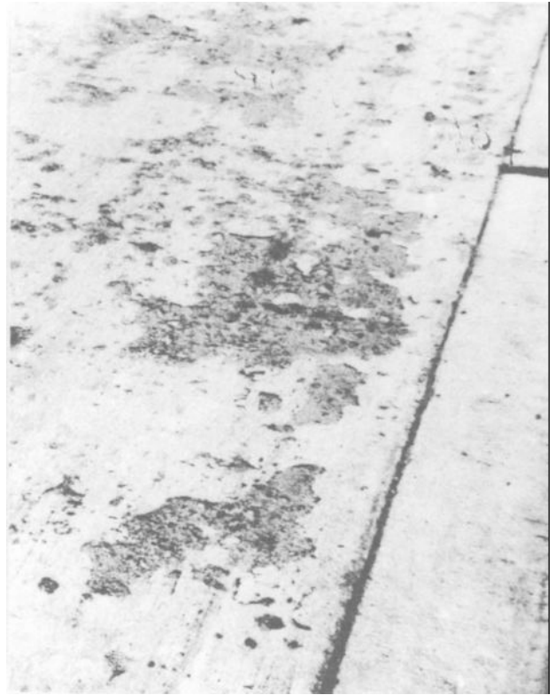
Figure 5-4. Light scale.
