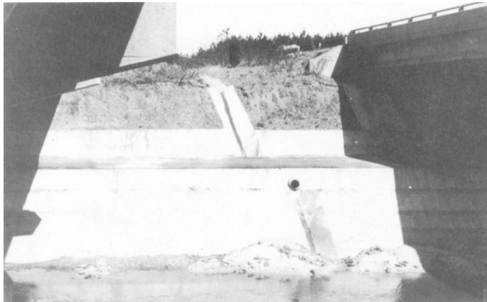
Figure 5-38. Concrete slope protection.
