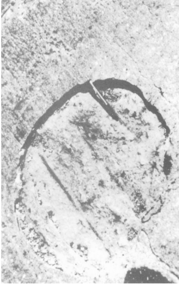
Figure 5-8. Large spall.
