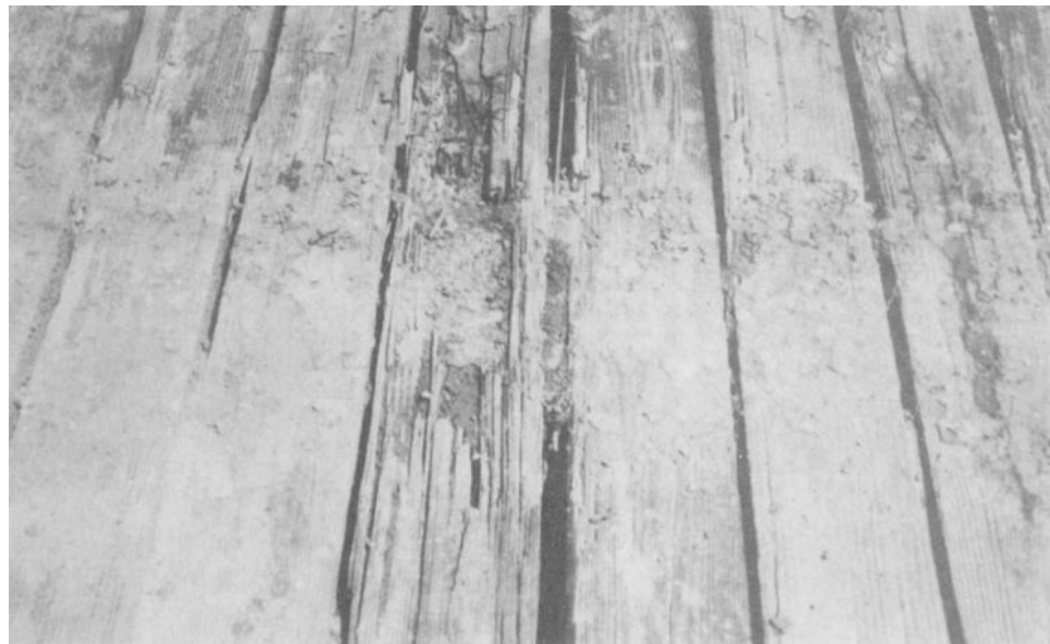
Figure 5-16. Slight and advanced wear on a timber deck (mechanical abrasion wear also present).
