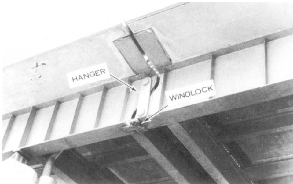
Figure 3-14. Pin and hanger connection.
