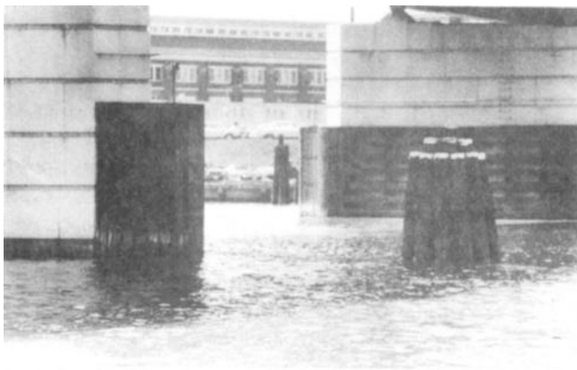
Figure 3-18. Timber pile cluster dolphins and timber fenders.
