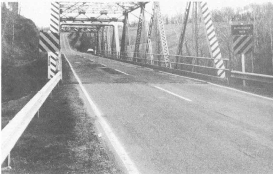
Figure 8-35. Appropriate markings for clearances on civilian bridges.
