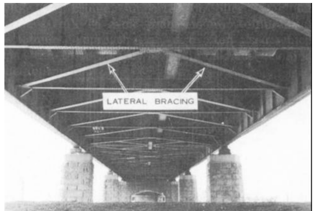
Figure 3-9. Bracing. (Sheet 2 of 2)
