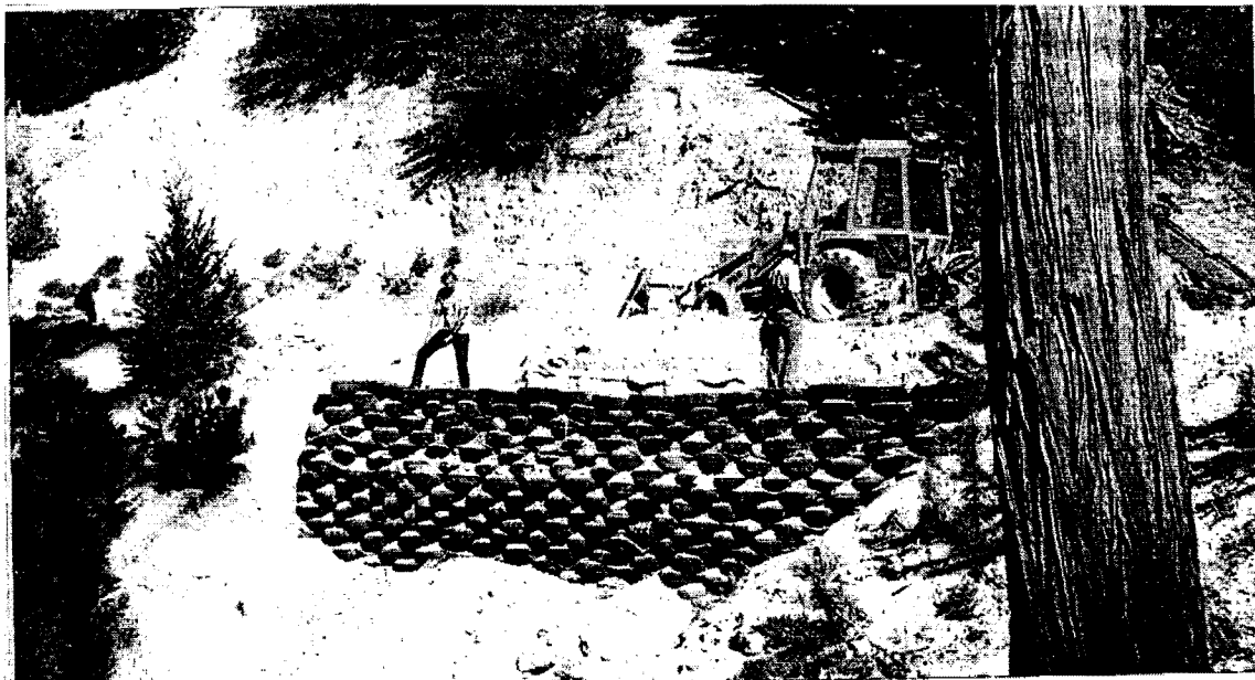
Figure 2.4. A Tire-faced Wall in California (7)
