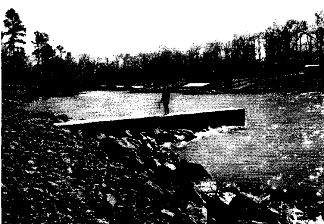
Figure 2.14: River Wing Dam Built Using Eco-Blocs (10)
