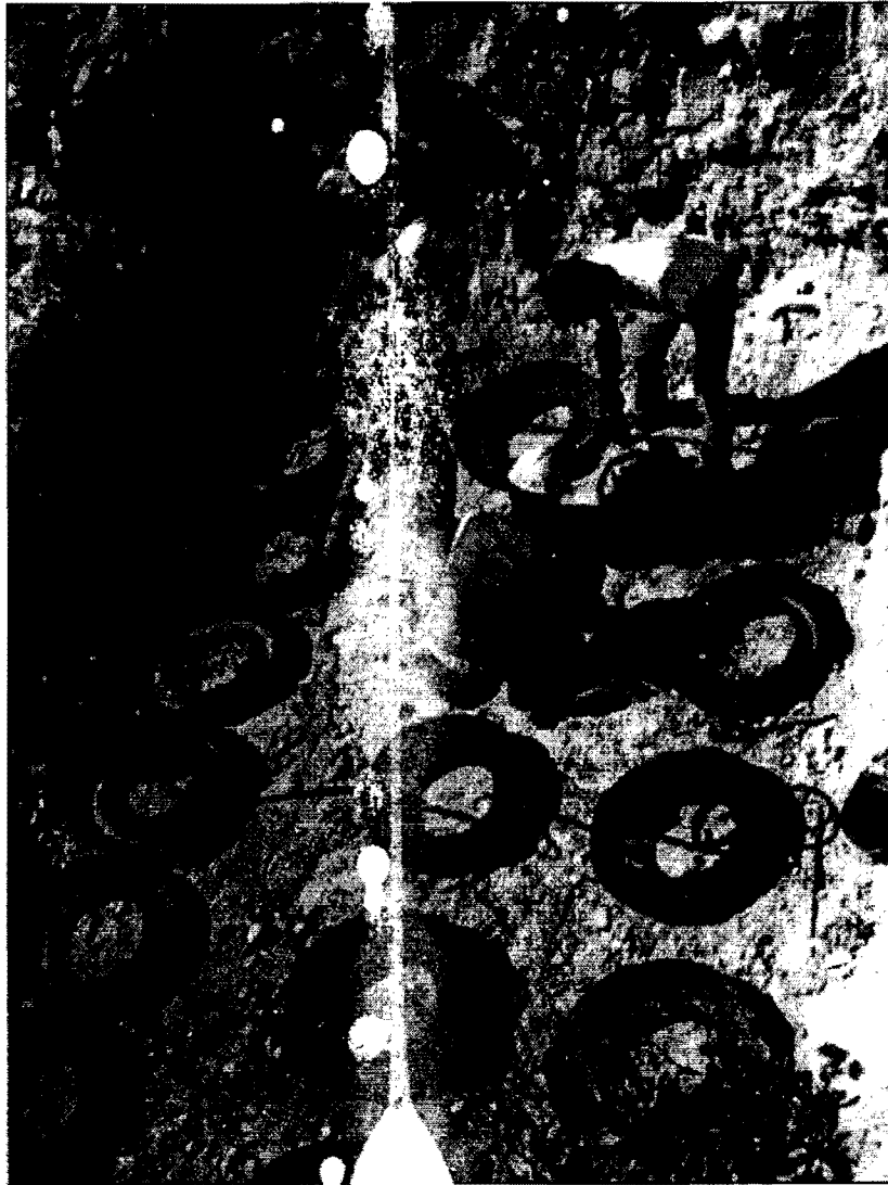
Figure 2.6. Tire Halves Tied with Rope (14)
