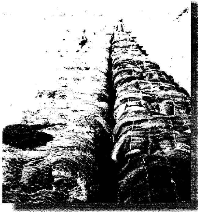
Figure 2.20: Bales on top of Concrete Foundation (12)
