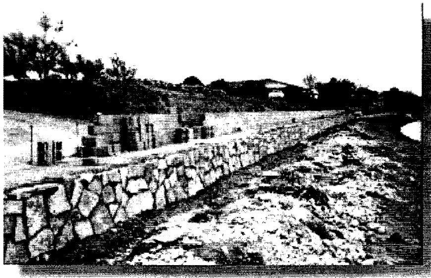
Figure 2.22: Block Retaining Wall on Top of Bales (12)
