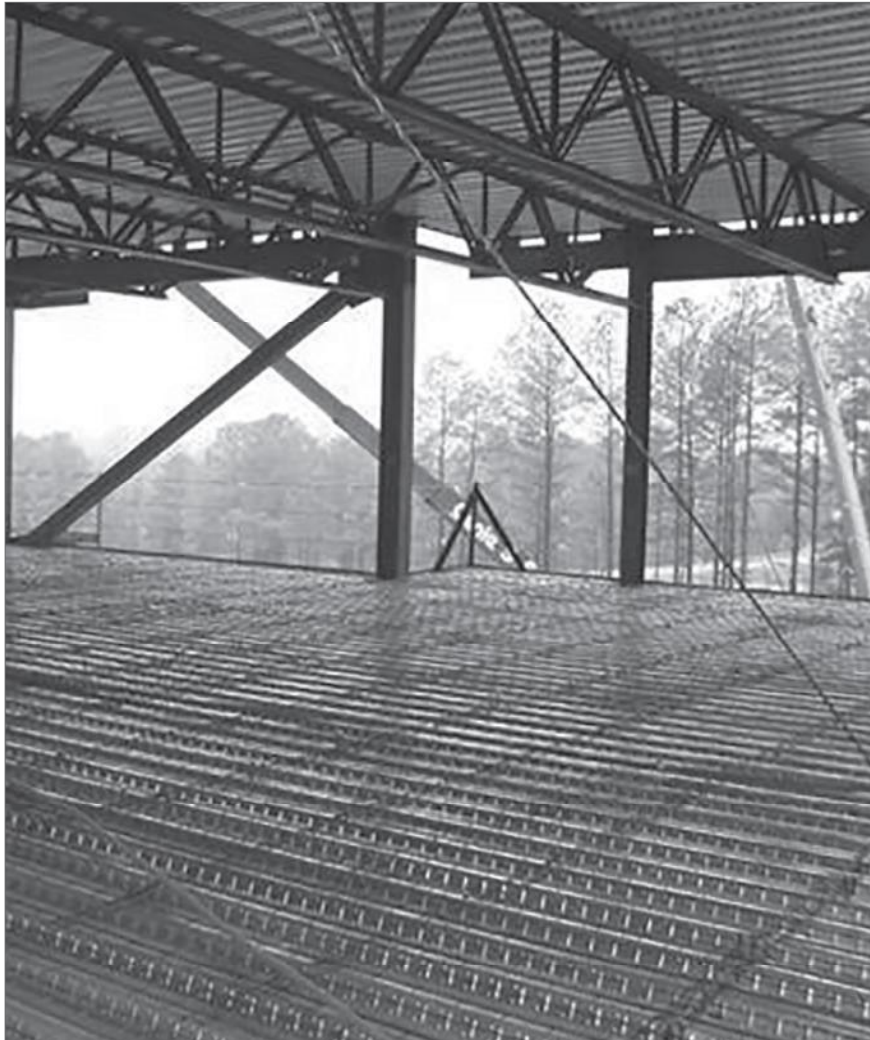
A typical steel deck installation.
