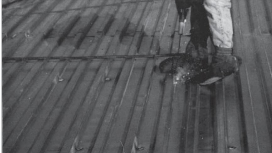
Fastening steel deck by welding.
