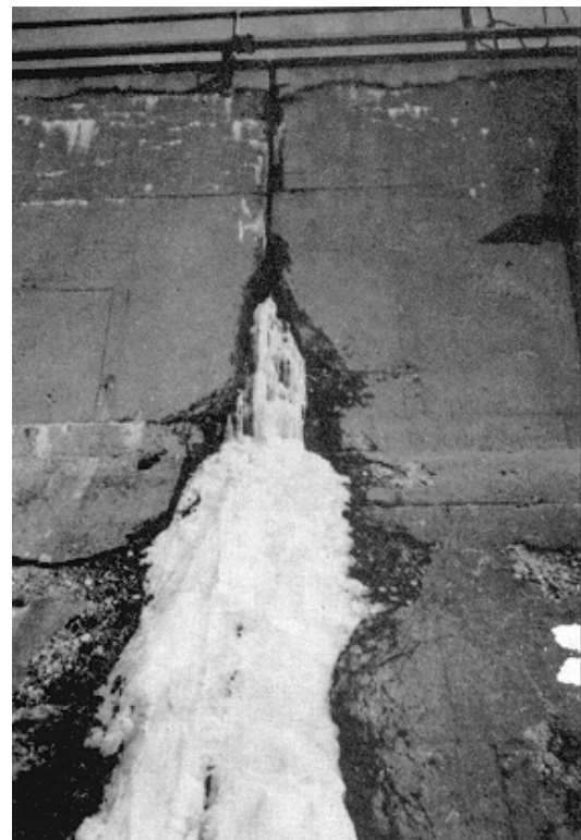
Figure 2-28. Water seepage through joint
