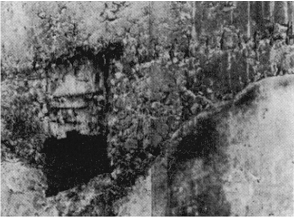
Figure 2-2. Honeycombing and cold joint
