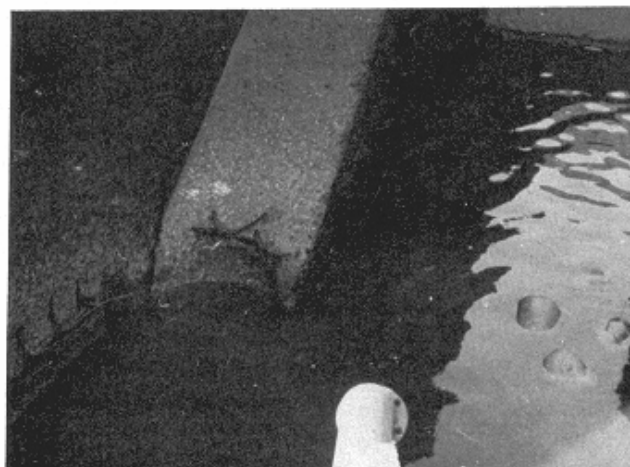
b. Erosion behind wall baffle
