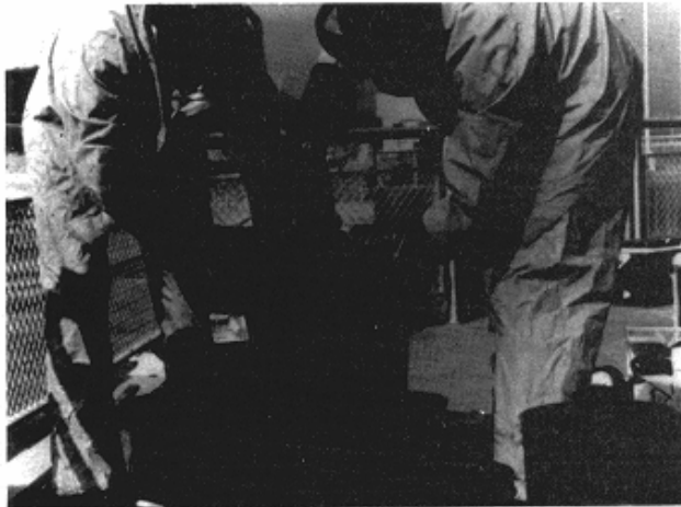
a. Saturating burlap bags with chemical grout
