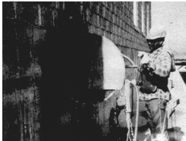
Figure 5-3. Diamond-blade saw
