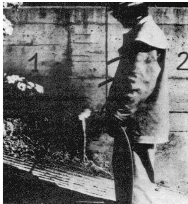
Figure 5-6. Thermal lance
