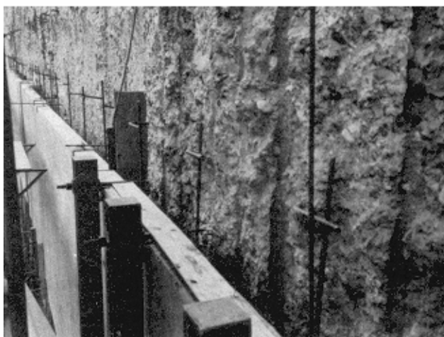
Figure 8-15. Installation of precast concrete stay-in-place forms at Troy Lock, Hudson River (Miles 1993)
