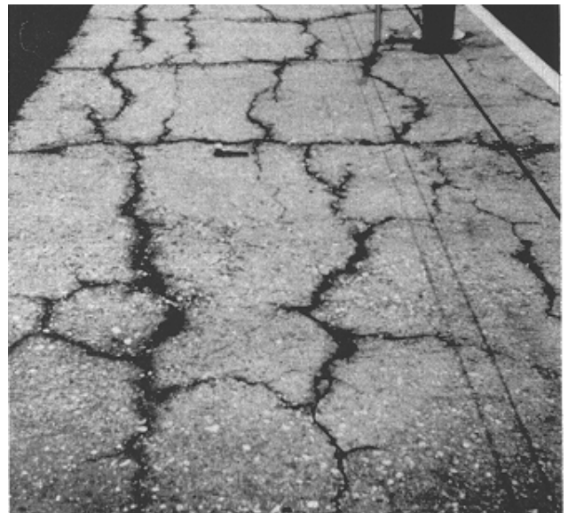
Figure 2-6. Pattern cracking resulting from alkali-silica reaction
